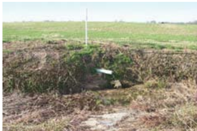
This outlet pipe is a sign of drain tile located in this field. Removal of drain tile is fairly simple, and outlets such as these are subsequently plugged.
